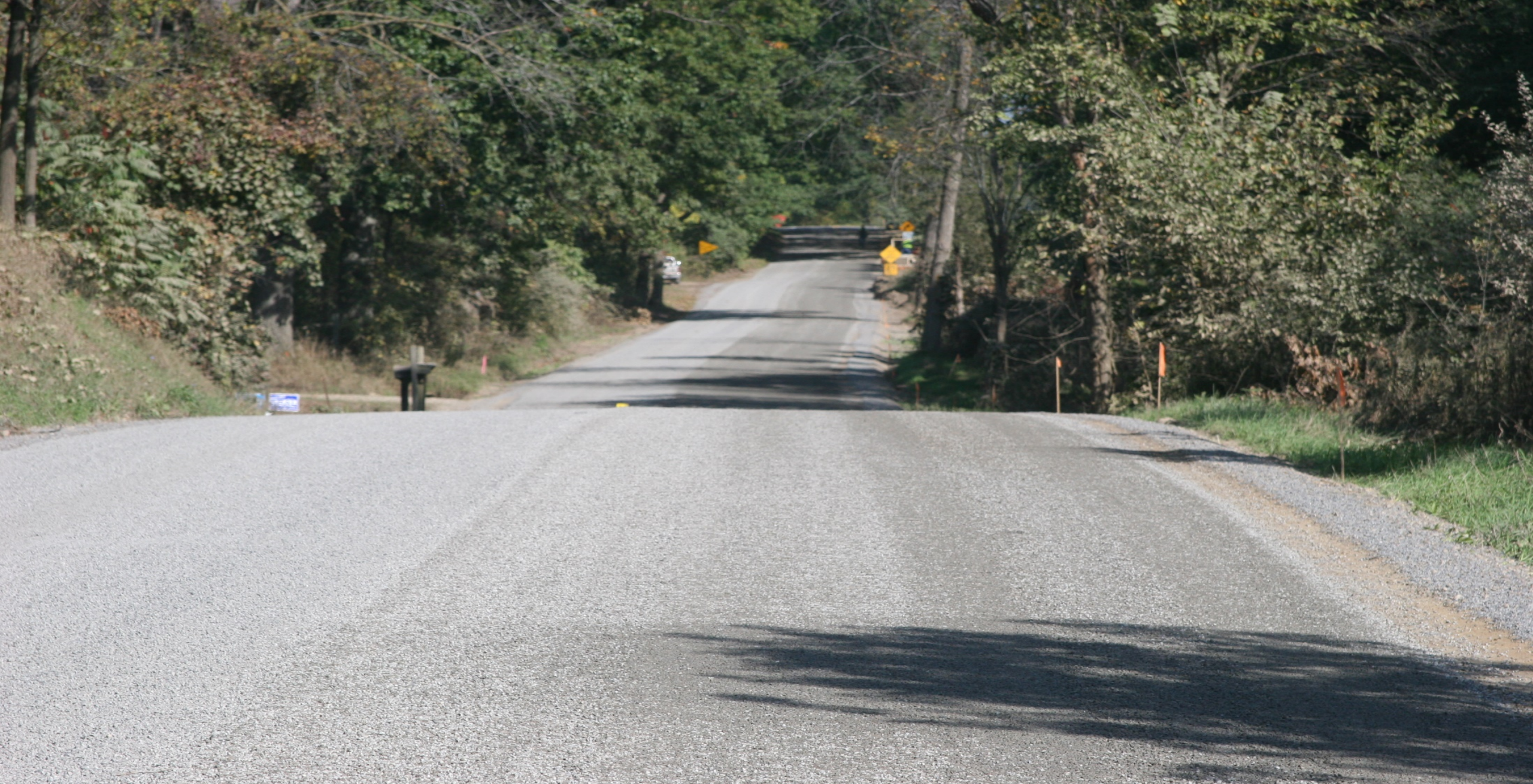
Secondary Road Reclamation Utilizing Sustainable Steel Slag Products
